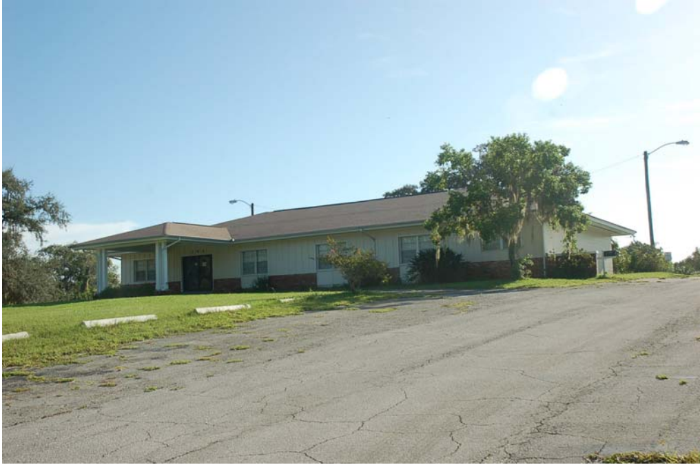
View looking south from Singleton Avenue at the north and west elevations.
