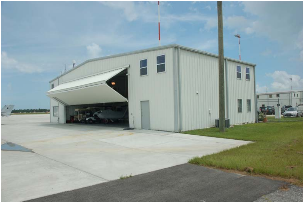
View of the south and west elevations.
