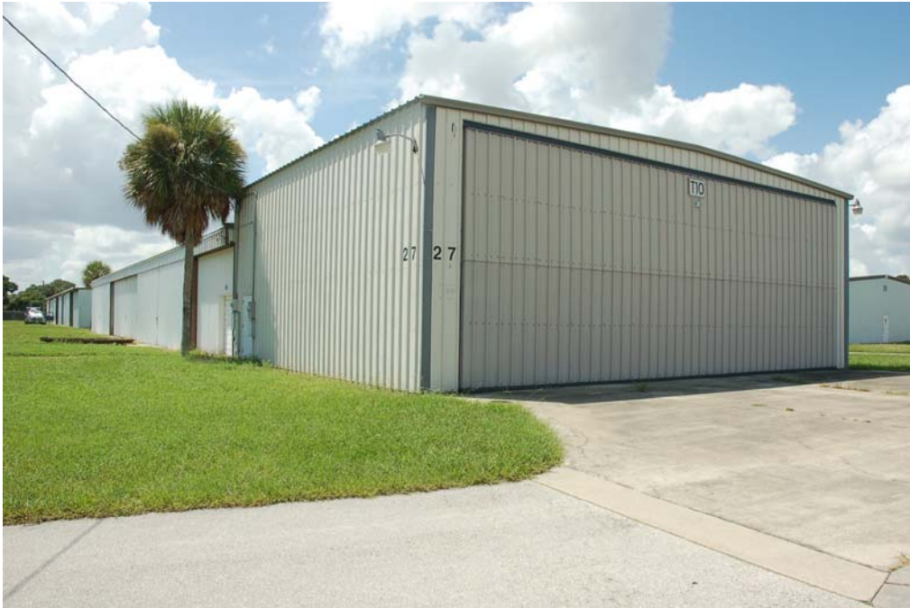
View of north and east elevations.
