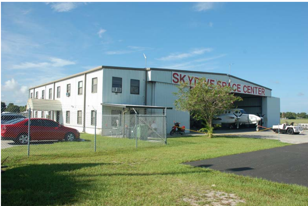
View of north and east elevations.
