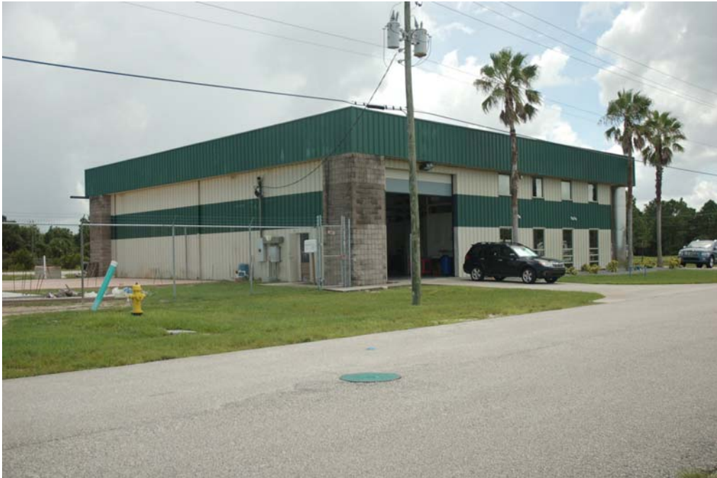
View of the north and west elevations.
