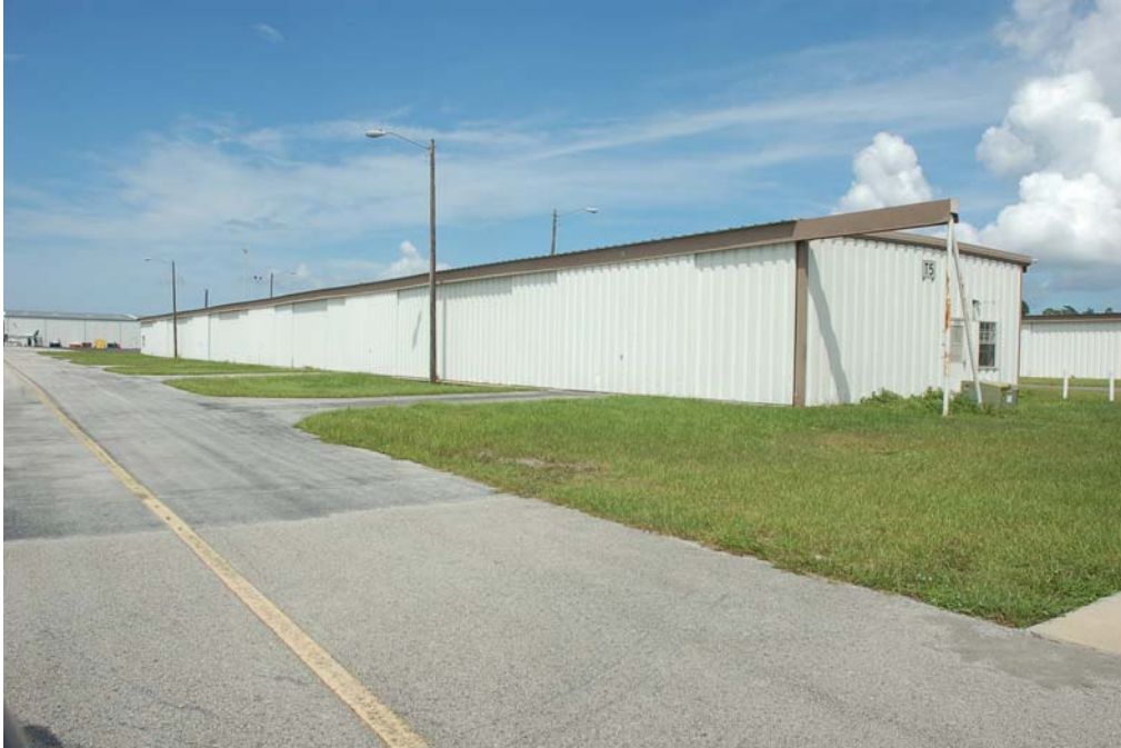
View of the south and west elevations.
