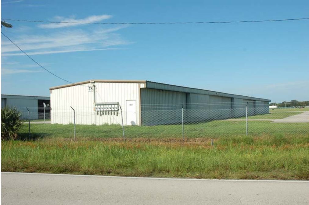
View of the north and east elevations.
