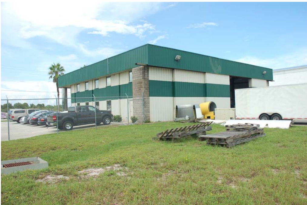
View of the south and east elevations.
