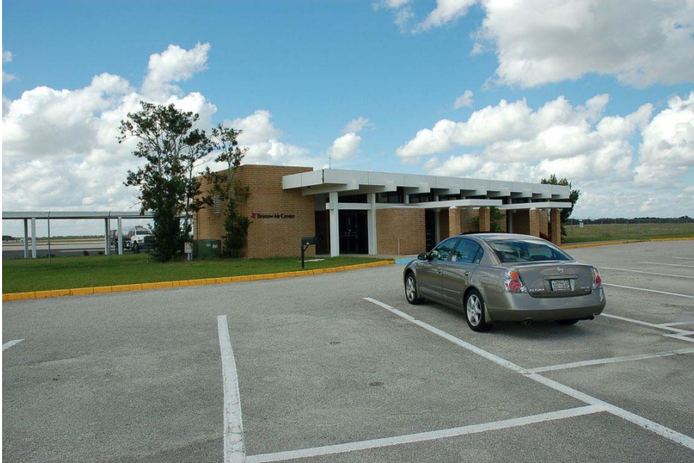
View of the south and east elevations.
