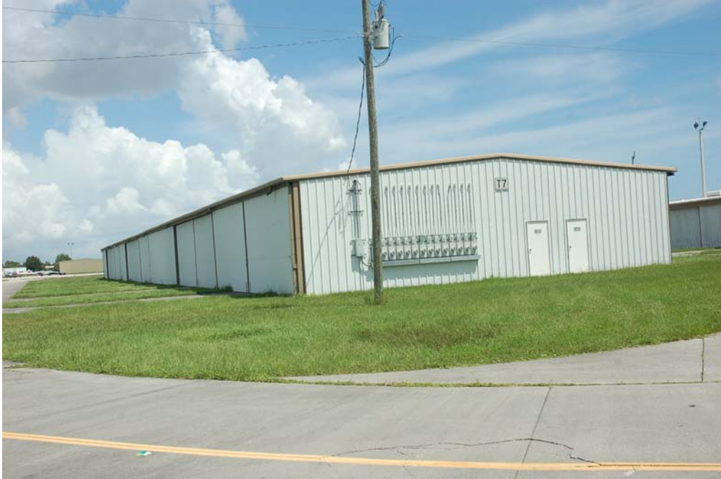
View of the south and west elevations.
