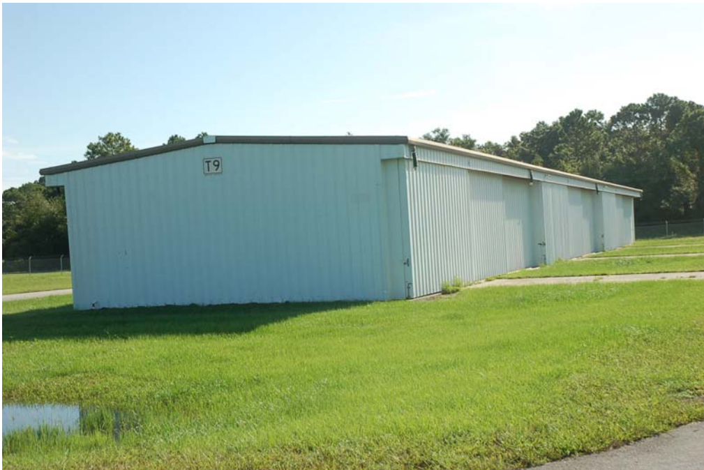
View of the south and west elevations.
