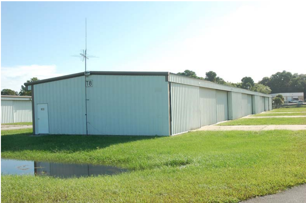
View of the south and west elevations.
