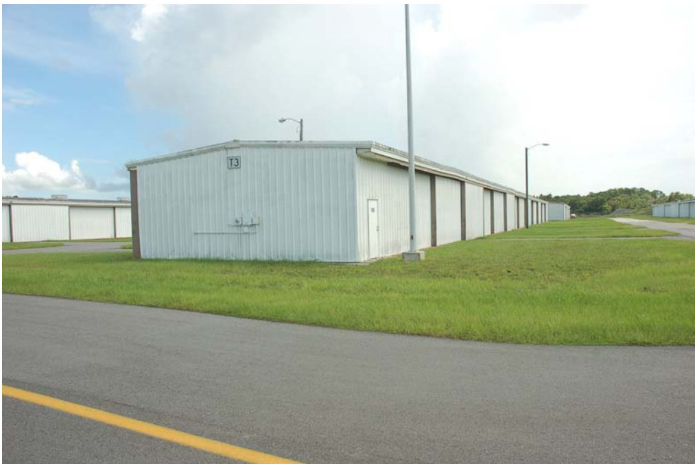
View of the north and west elevations.
