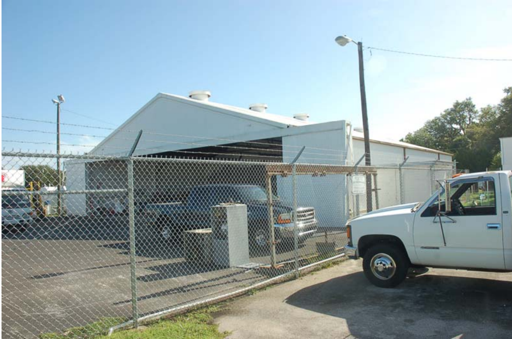
View of the south and west elevations.
