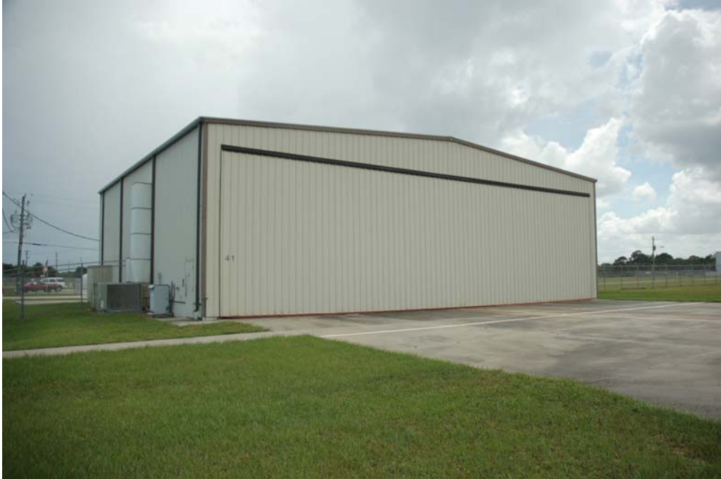
View of the north and west elevations.
