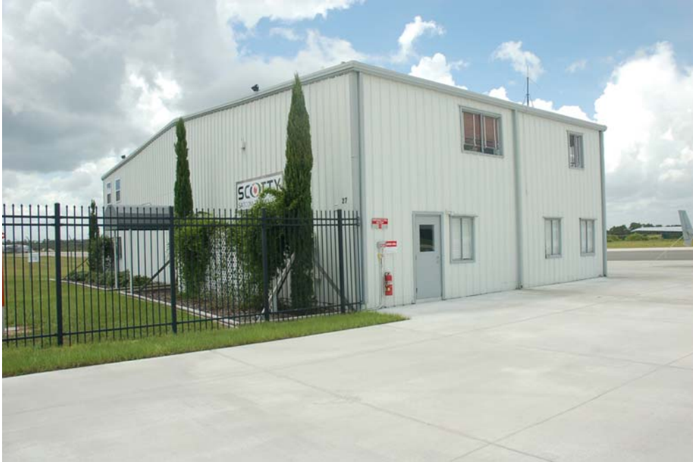
View of the north and east elevations.
