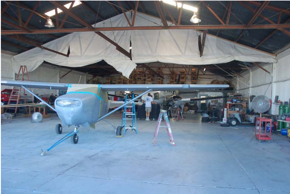
Interior view of the hangar area.
