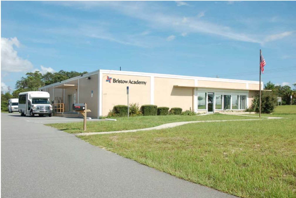
View looking southeast from Tico Road of the north and west elevations.
