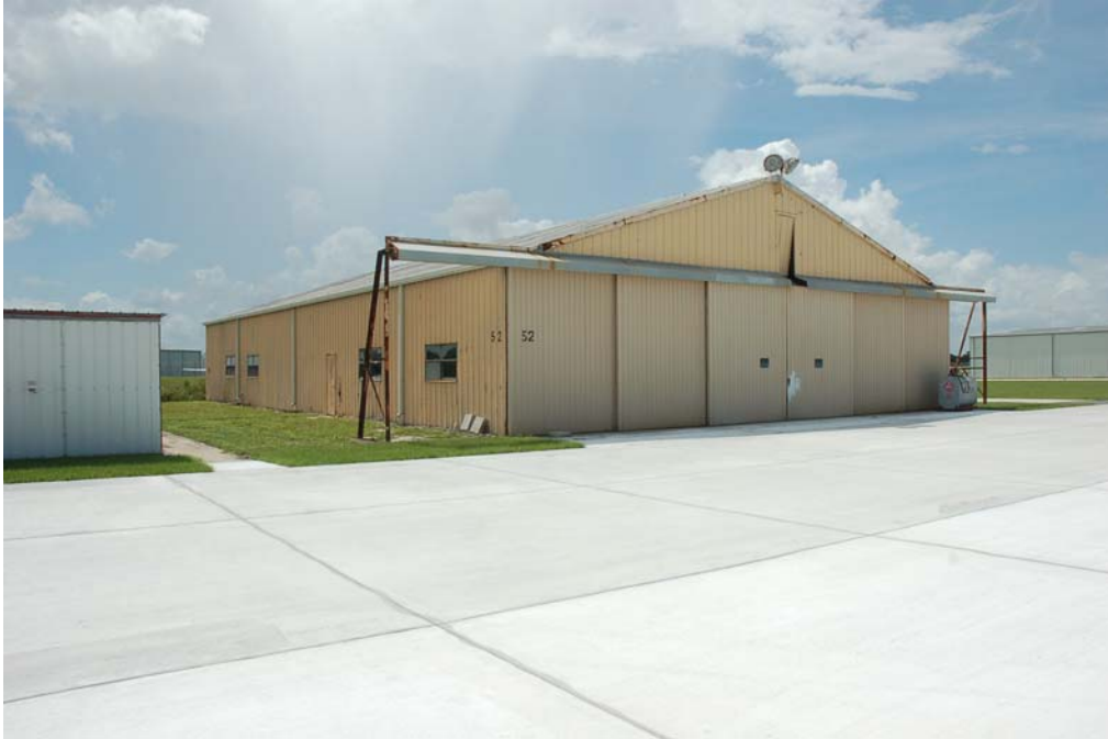
View of the north and west elevations.
