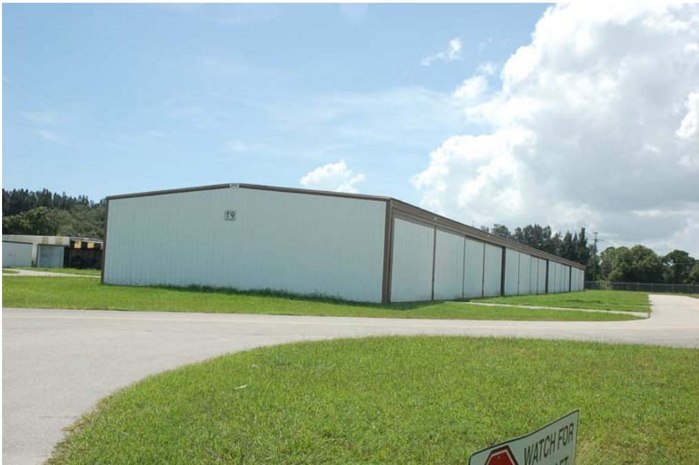
View of the north and west elevations.
