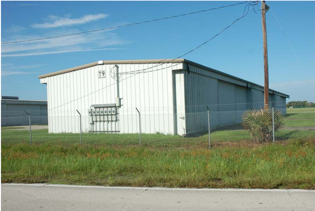
View of the north and east elevations.
