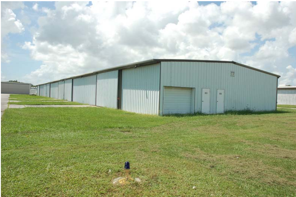
View of the north and east elevations.
