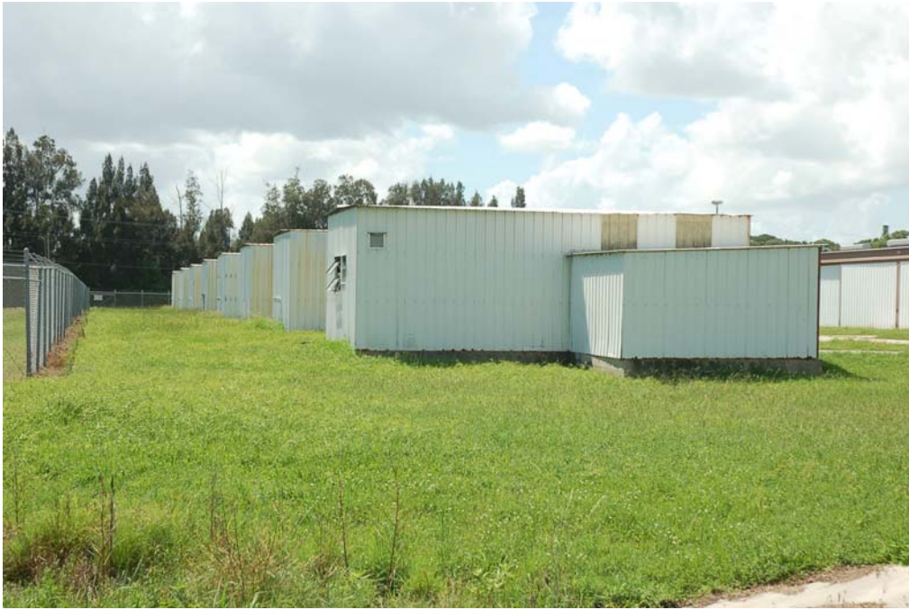
View of the north and west elevations.
