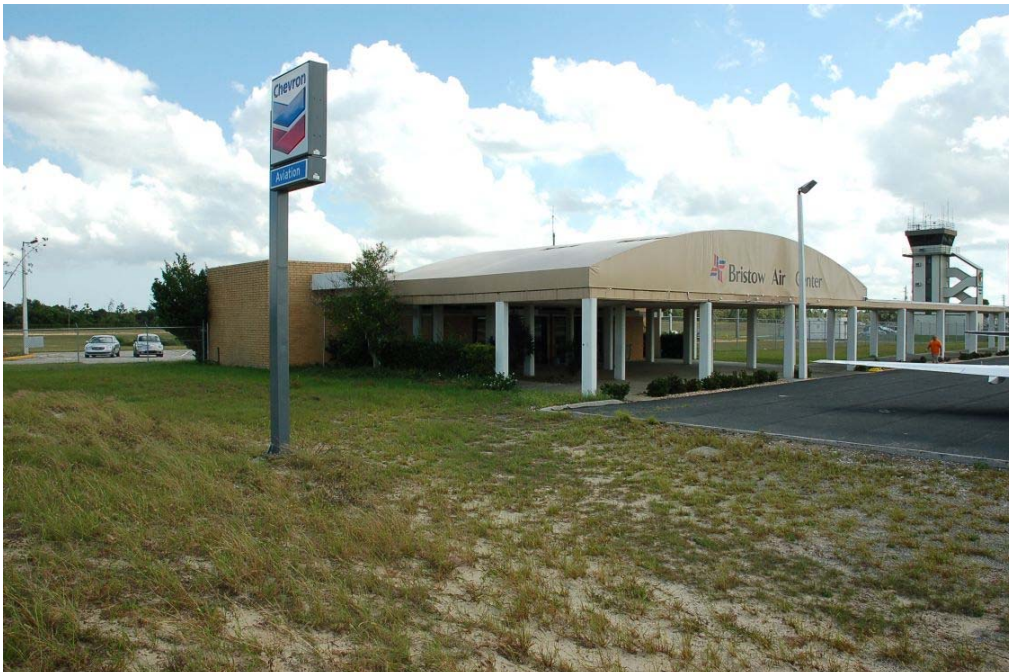
View of the north and west elevations.
