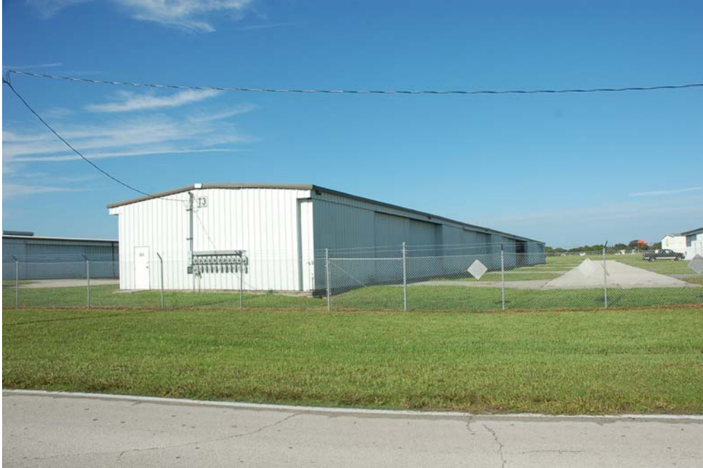
View of the north and east elevations.
