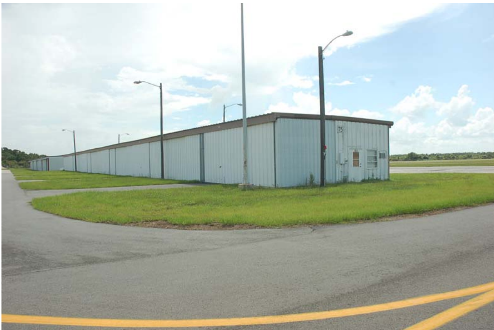
View of the north and east elevations.
