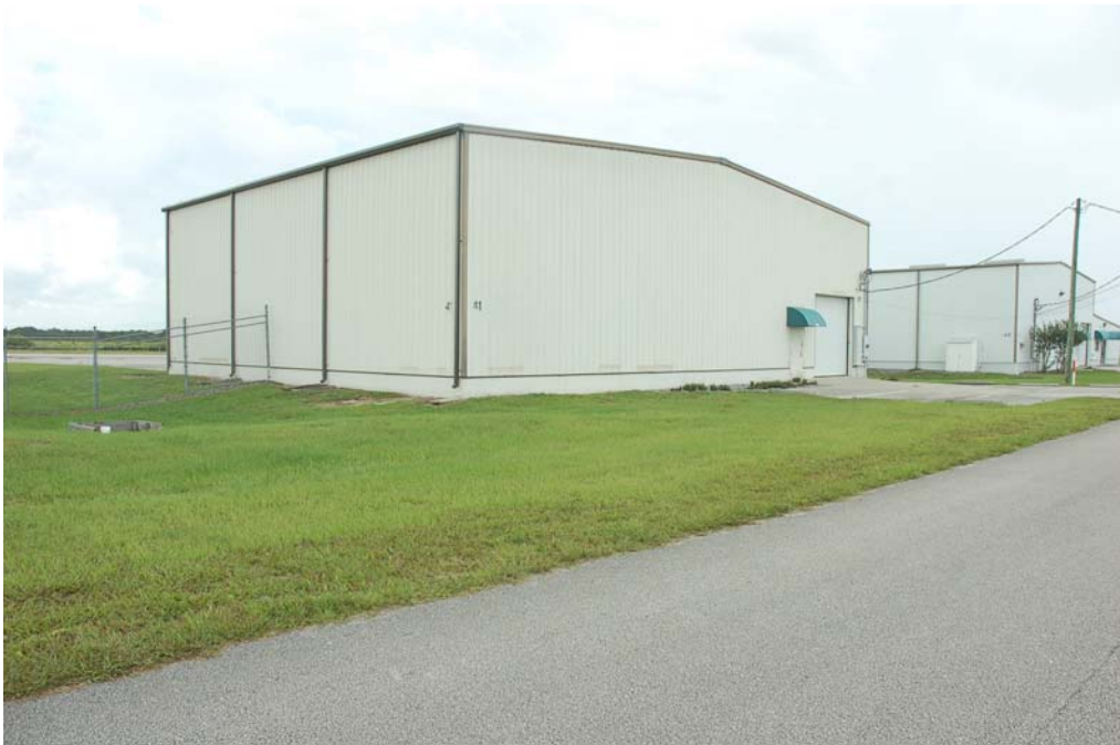
View of the south and east elevations.
