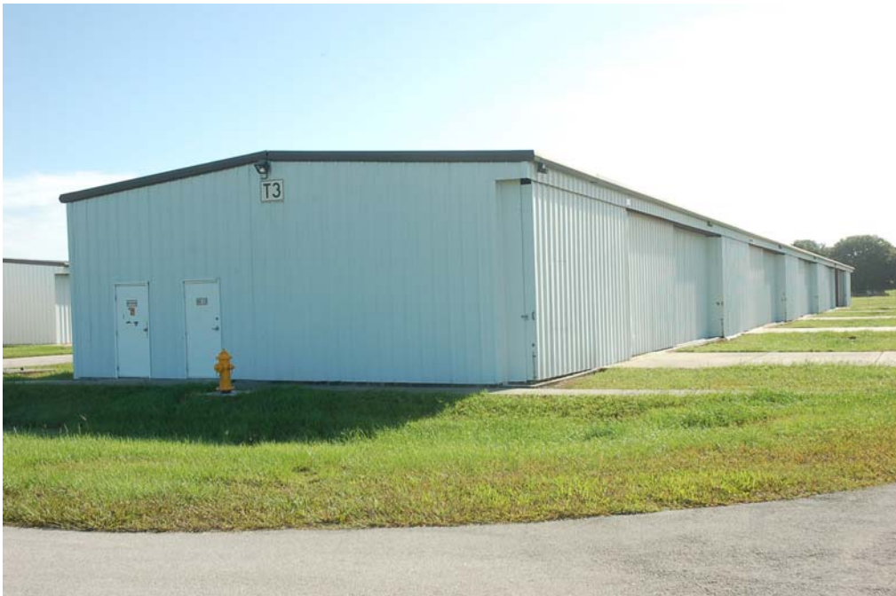
View of the south and west elevations.
